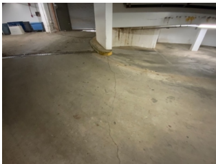
Concrete Parking Lot
