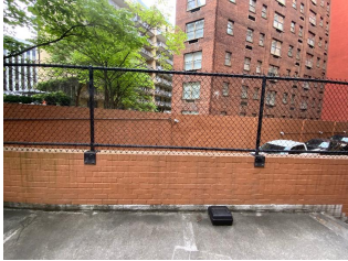
Chain Link Fencing
