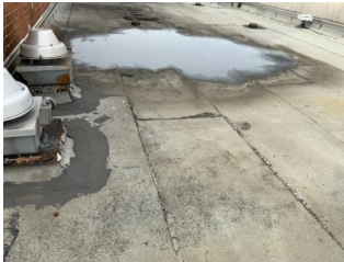
Modified Bitumen Roof
