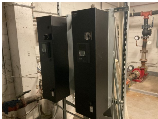
Variable Frequency Drive - 20 HP -3
