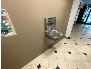
Water Coolers - Wall-Mounted
