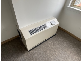
Heat Pump - Water Source
