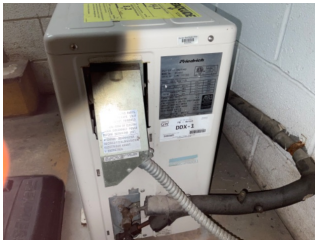
Split System Heat Pump - 3/4 Ton
