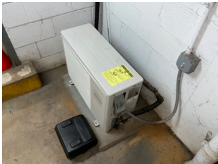
Split System Heat Pump - 3/4 Ton
