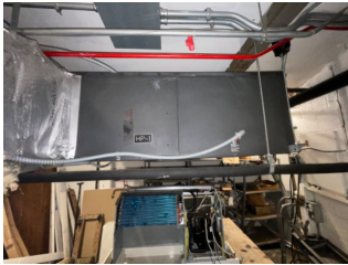
Heat Pump - Water Source
