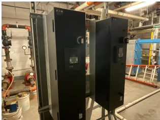
Variable Frequency Drive - 20 HP -4
