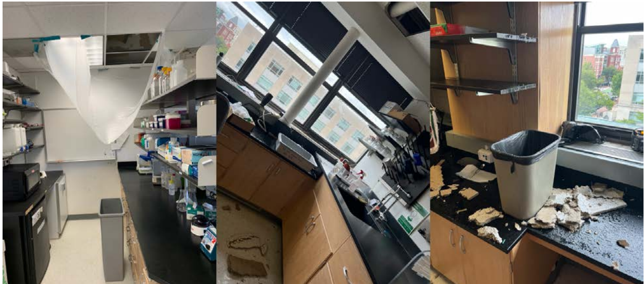
Appendix 8. Fallen ceiling tiles and leaks due to demolition of the 5 th floor greenhouse
